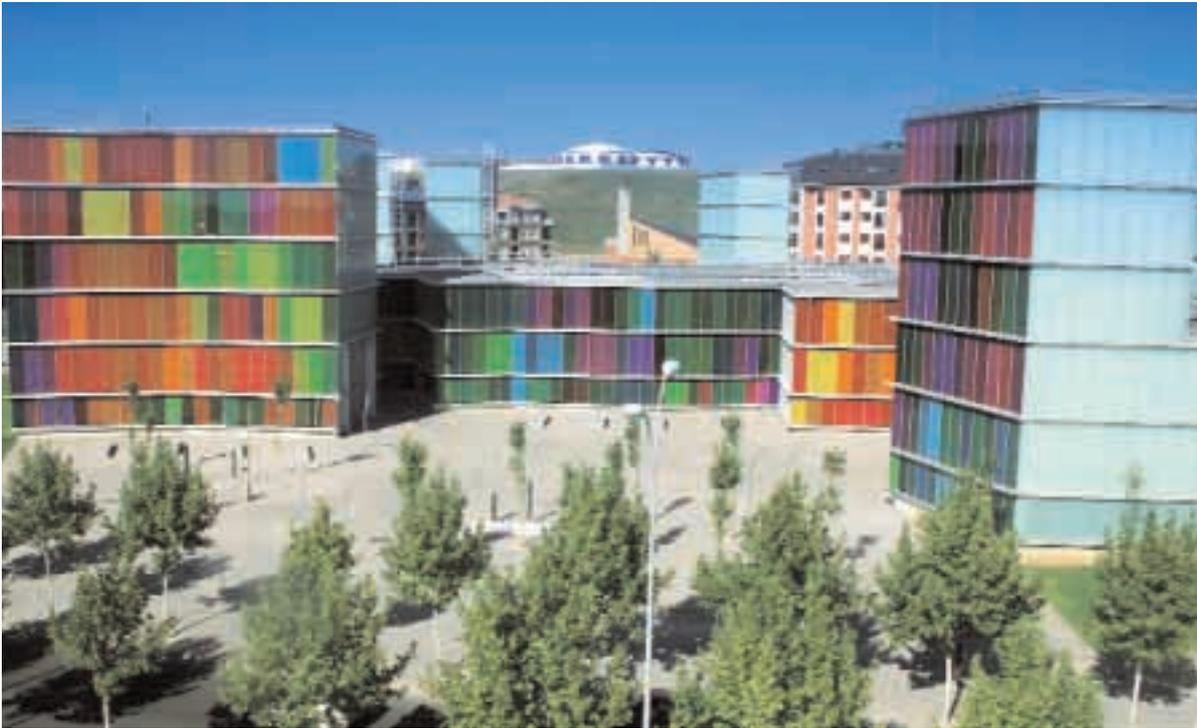
Its main facade consists of more than 3,300 multi-coloured glass panes held together by more than 500 iron beams. The design takes its inspiration from the oldest stained glass window in the Cathedral of León, known as "The Falconer", dating back to the twelfth century. The building also has two types of roofing, an inverted gravel structure, and another ventilated ceiling made of zinc.
